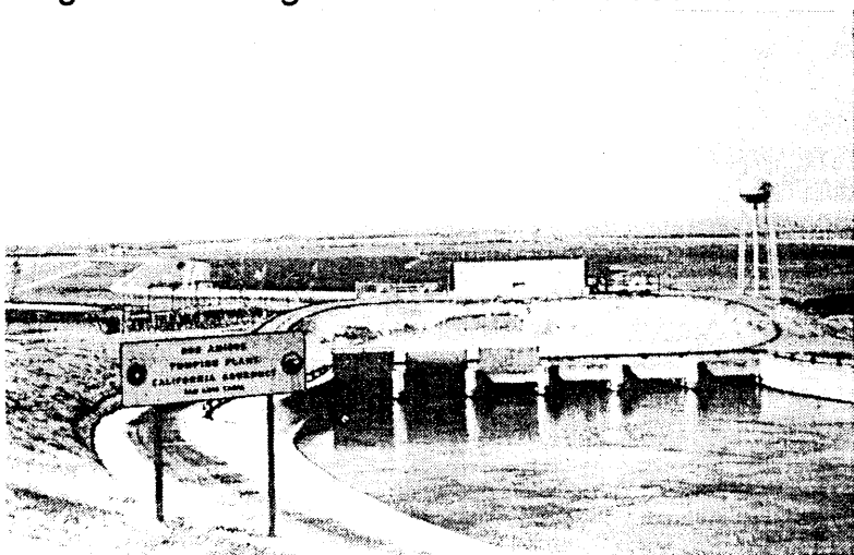
Figure 1. California Aqueduct; Dos Amigos Pumping Plant lifts water from Reach 3 to Reach 4
